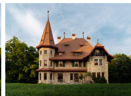
M.A.D House Exterior view
