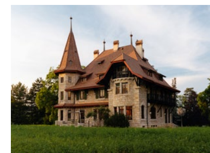
M.A.D House Exterior view
