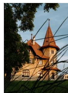
M.A.D House Exterior view
